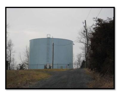
storage tank containing 500,000 gallons storage. This tank was brought on line in 1969 and has been in continuous service.
